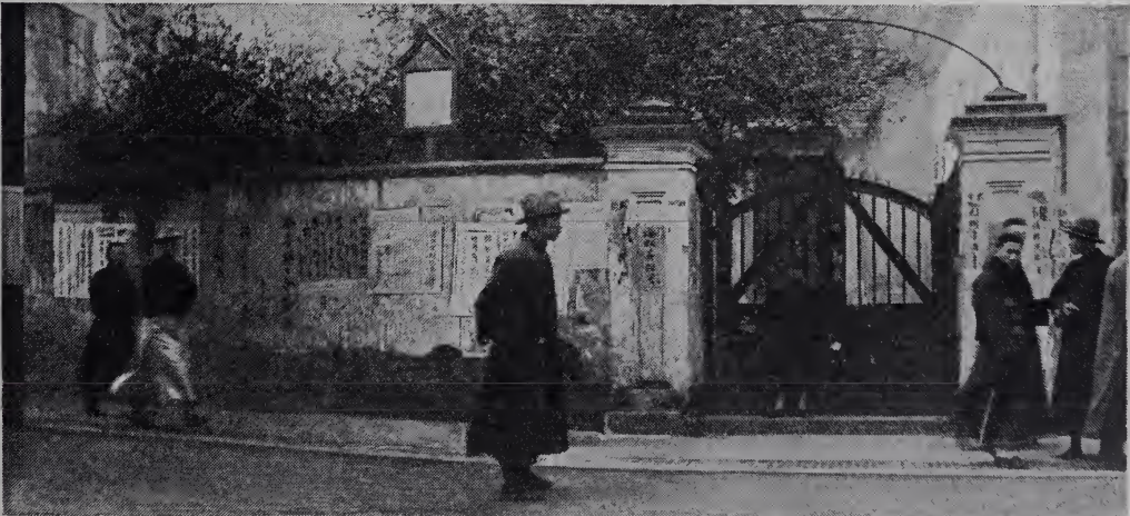
A Christian Church of China in Hankow. Formerly the L.M.S. Church. Walls plastered with posters "Down with Christianity" etc. Full congregations inside
